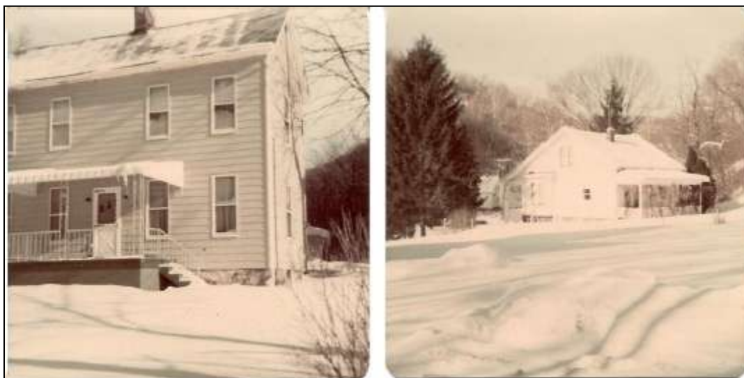
L - Home of Edward & Mildred Burke -- R - The Bell Home (rear). The picture of the Bell home was taken from the Burke property.
